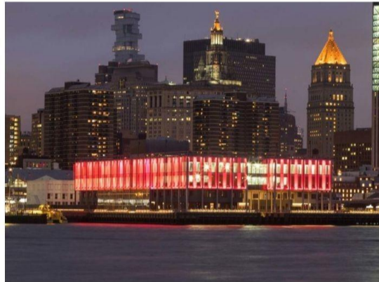
South Street, Pier 17,
